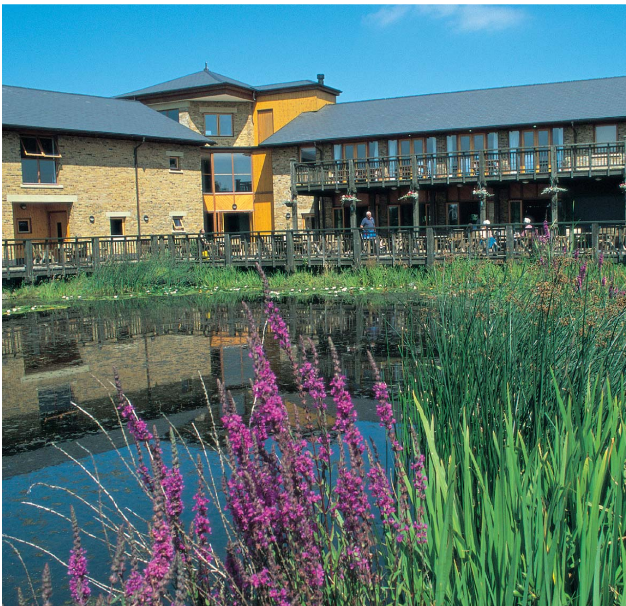
WWT London Wetland Centre
