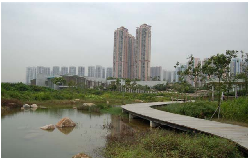
Photographie 3 – Ponton en bois au Hong Kong Wetland Park (© WWT with permission from AFCD, Hong Kong Government)
